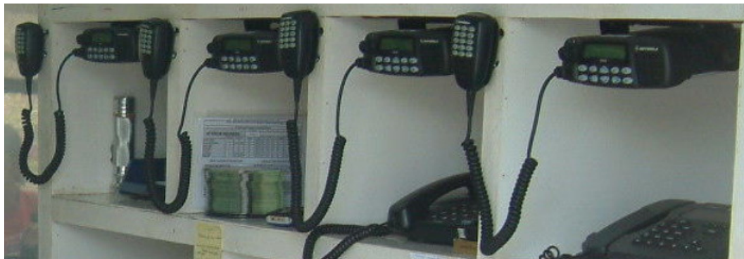
Multiple VHF base stations in a typical Inter Agency radio room monitoring a number of channels
