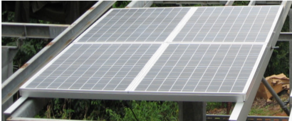
Solar panel array
