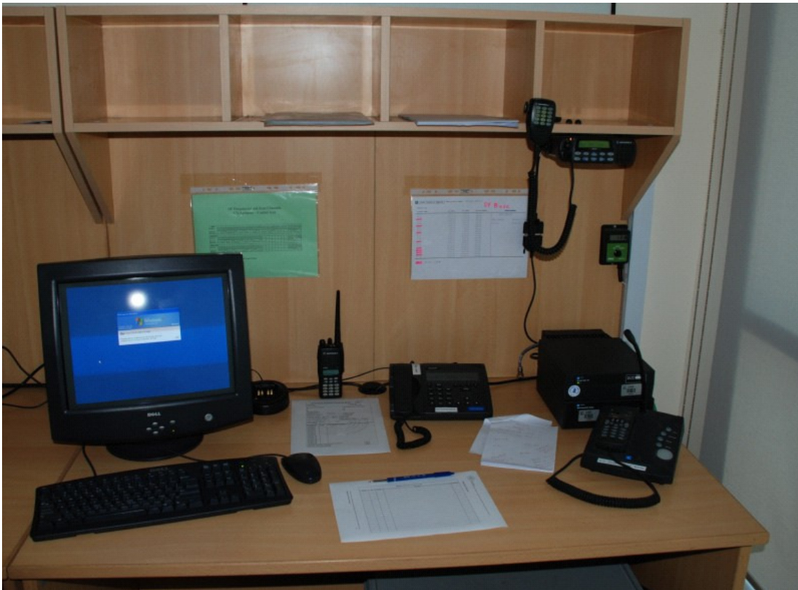
Example of a radio room setup
