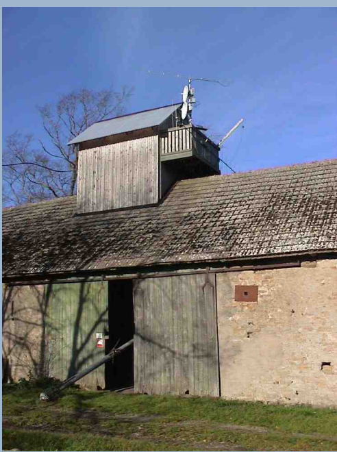
My antenna installation on a nearby barn.
